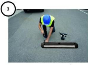
Asphalt : Fixing = Ø 11 x300mm
